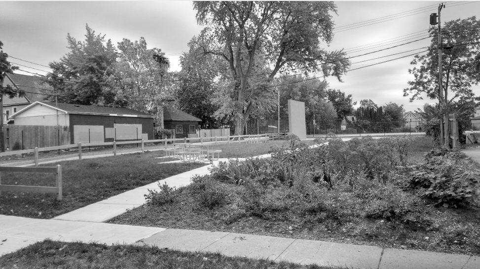
Figure 4-8b. (below) A handball court was constructed toward the rear of the parcel. In front are picnic tables and a gently sloping lawn that directs stormwater into a rain garden.
