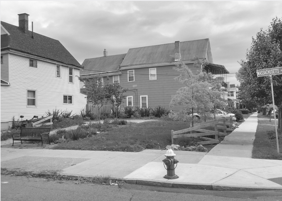
Figure 4-9b. (below) The completed corner park adds pervious off-street parking, a bench, and a small rain garden that collects stormwater from the roofs of two adjacent houses.
