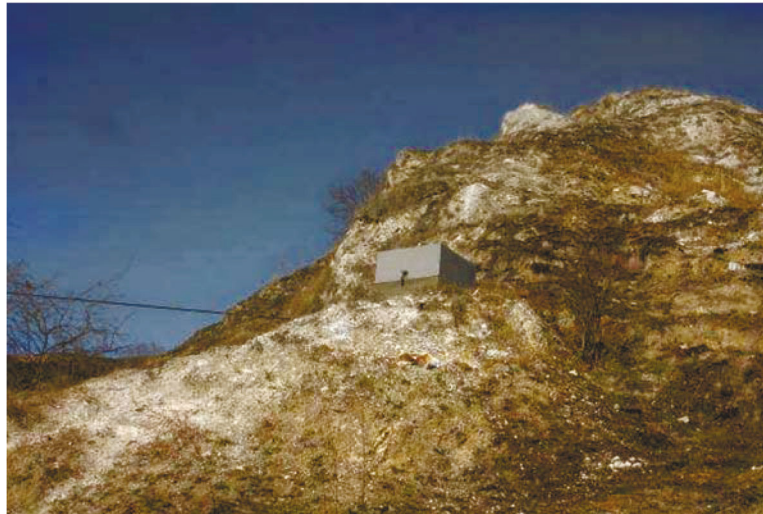
Fig. 5. General view of bunker encased in metal housing at Gornoye station.
