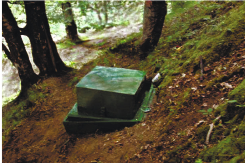
Fig. 4. General view of bunker encased in metal housing at Guzeripl station.
