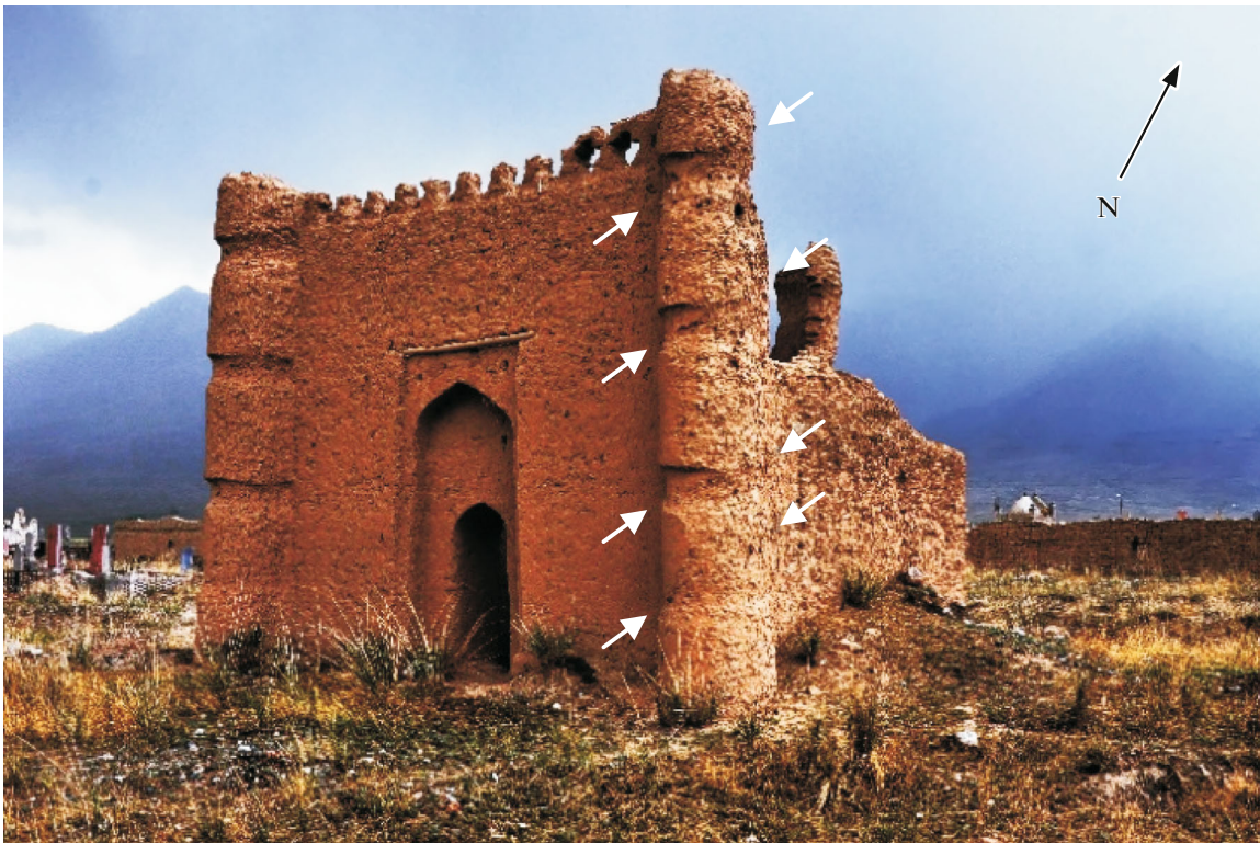
Fig. 8. Systematic oblique fissures (shown by arrows) are traces of ancient damage to northwestern column of grave monument, Konur-Oleng River (after (Korzhenkov et al., 2018a), with changes).
