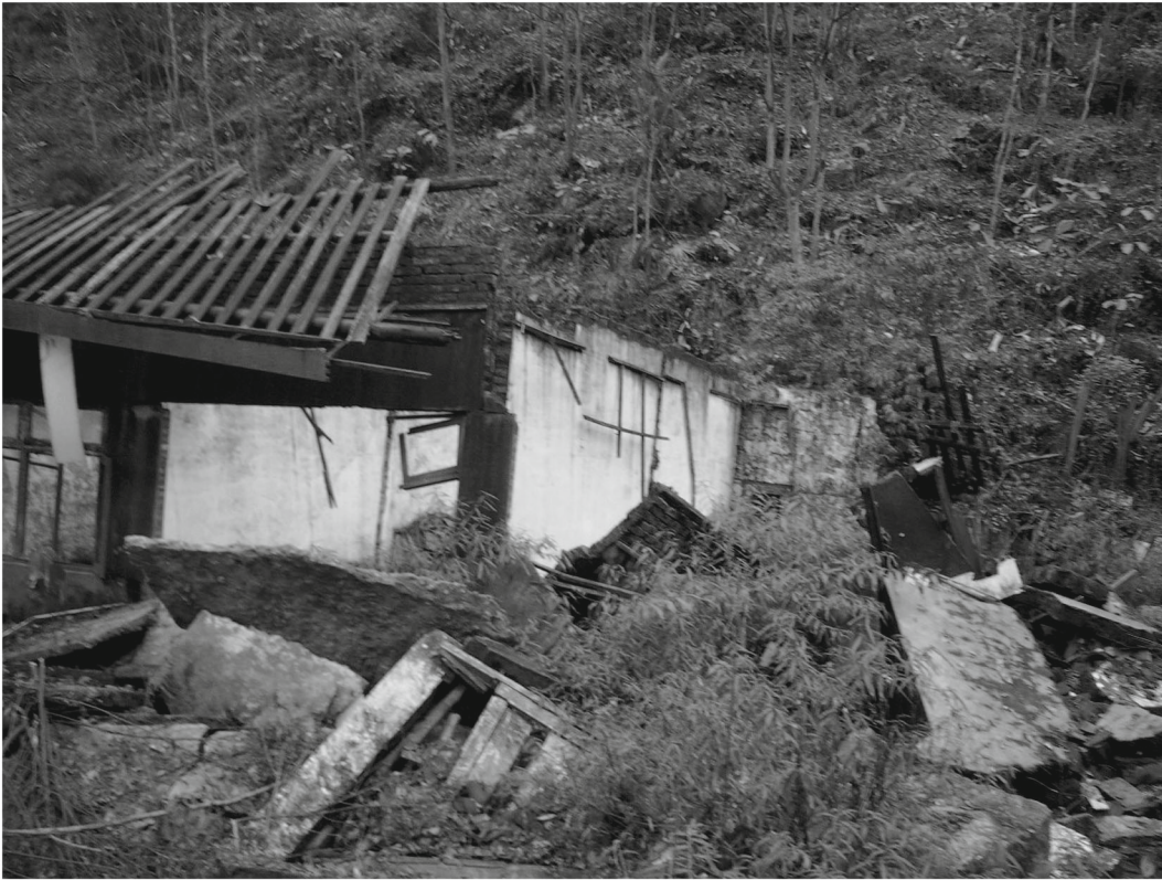
Fig. 9. Ruins of house in village of Hongkou after 2008 Wenchuan earthquake. Right-lateral strike-slip shifted back wall of house at foot of seismogenic scarp.
