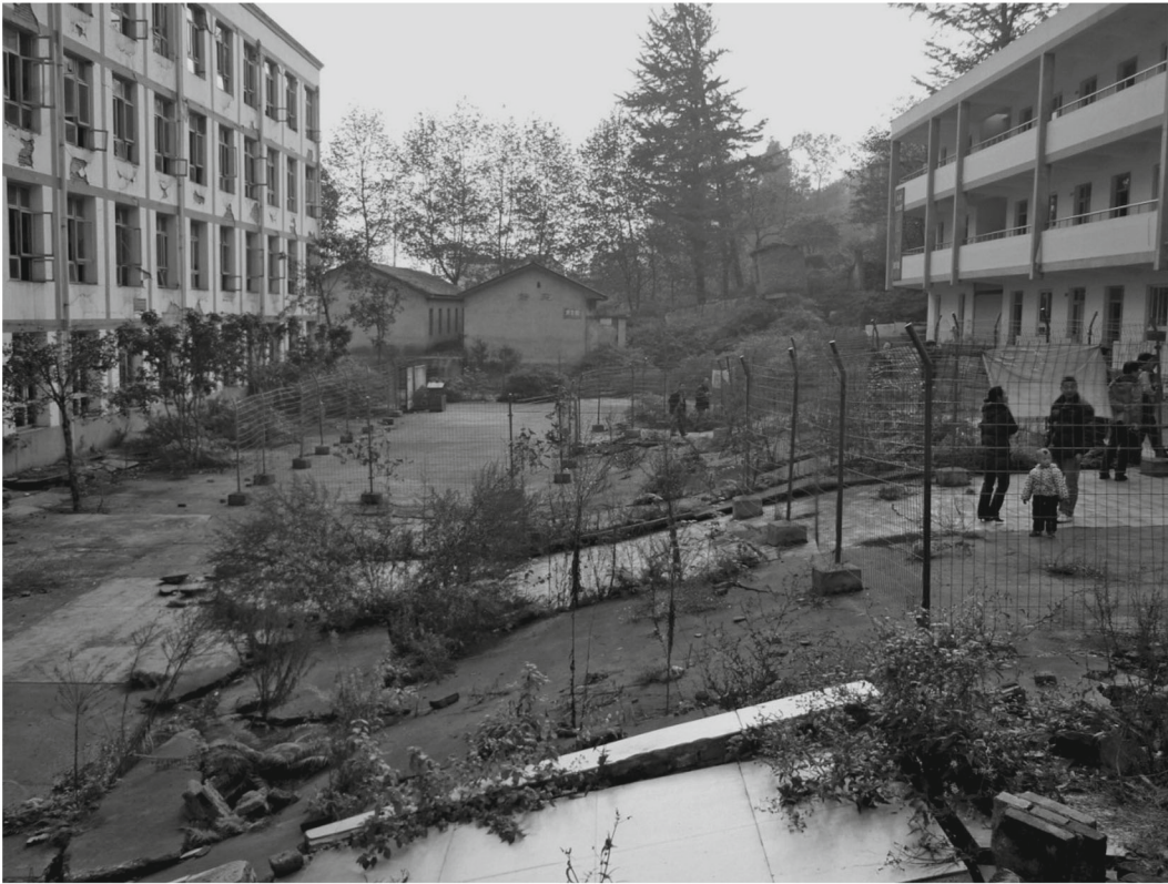
Fig. 7. Gently sloping scarp caused by 2008 Wenchuan earthquake, courtyard of Sino-French secondary school, Bailu.
