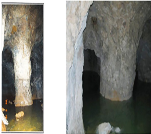
Fig. 18 Photo of pillar in the abandoned quarry with a thin layer of water at its base (by courtesy of Watelet JM, INERIS, France)
