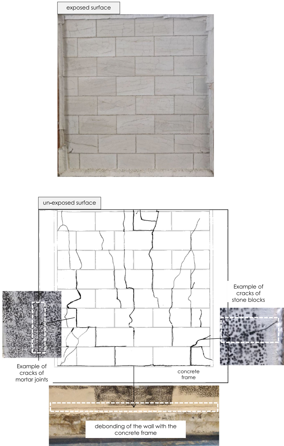
Fig. 10 Cracks on the exposed et un-exposed surface of the unloaded wall after the test
