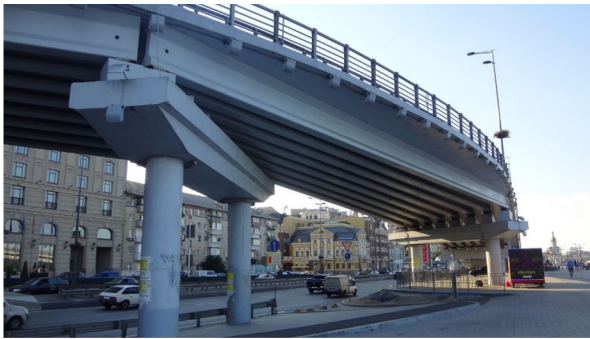
Fig. 1 Exemplary precast prestressed concrete bridge girders
