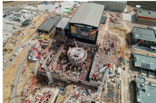
Figure 9. Bird's eye view of the ITER site in Cadarache with the growing torus hall in the middle; status: March 2018 (courtesy: ITER Organization/EJF Riche; more photos available under: https://www.iter.org/album/Media/4%20-%20Aerial ).
