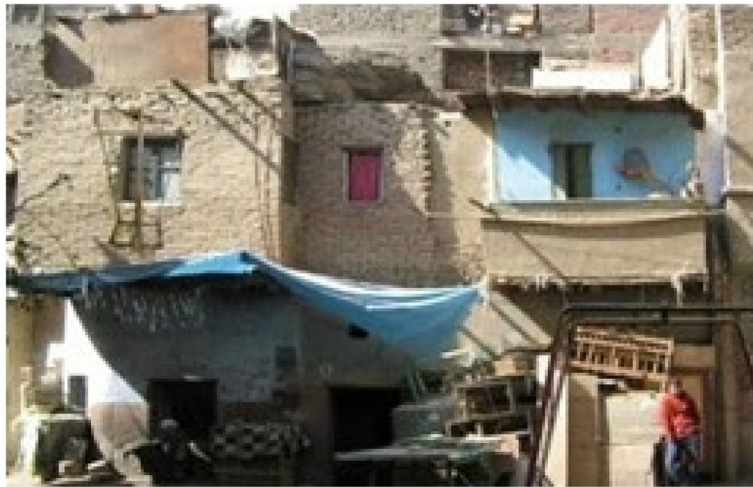
Fig. 12 Building facades before development [32]
