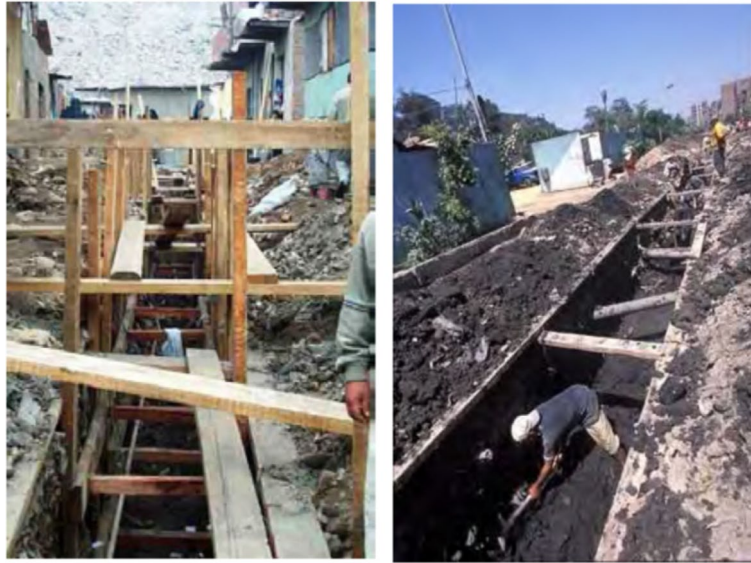
Fig. 14 Infrastructure interventions: improving the sewage network [31]
