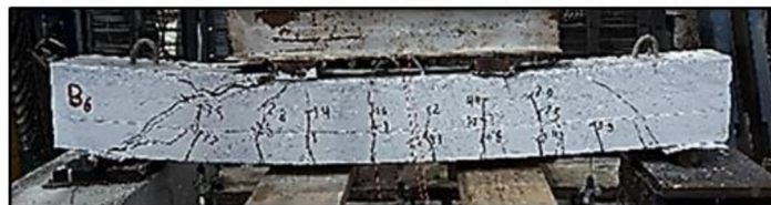
f: Crack Patterns at Failure load 34.05 ton for Tested Beam (B6)
