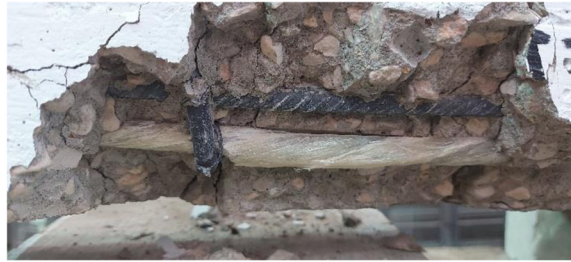
Fig. 7 Rupture of the GFRP bar at the failure of a tested beam specimen
