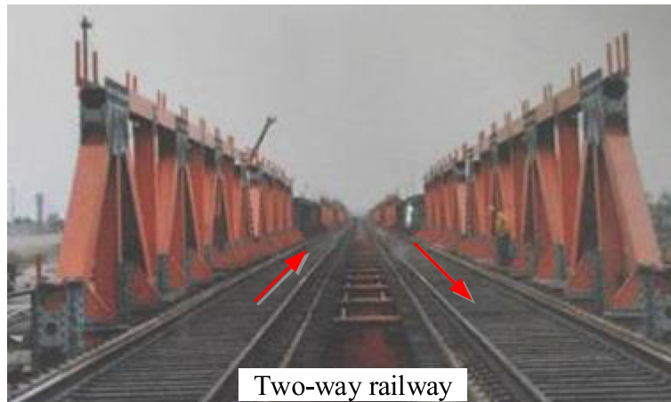
Fig. 5 'New' LuGou Railway Bridge in 1988
