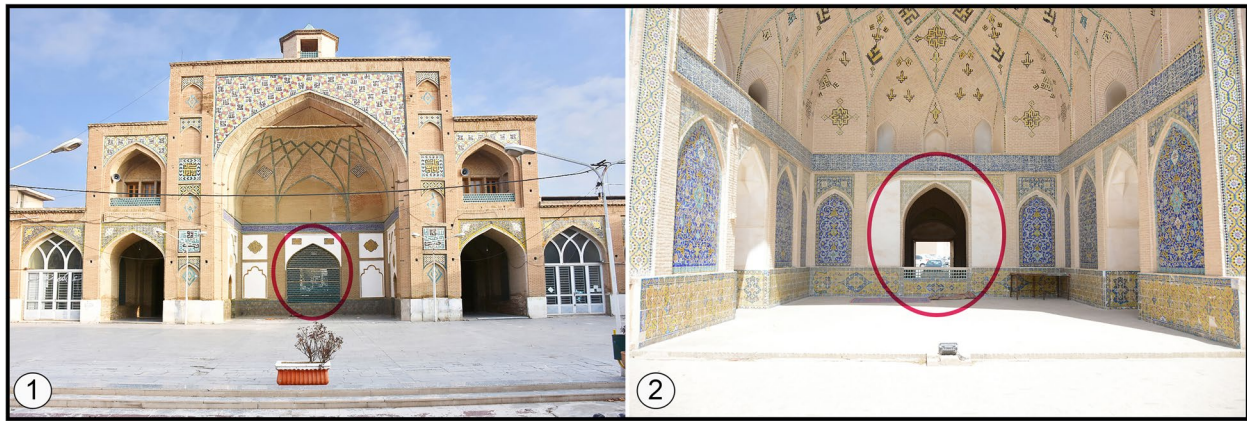
Fig. 11 1- The porous tile work (Fakhr and Madin) of the north iwan of the Sultani Mosque of Borujerd, 2- The opening of the north iwan of the Sultani Mosque of Semnan (Source: the authors)
