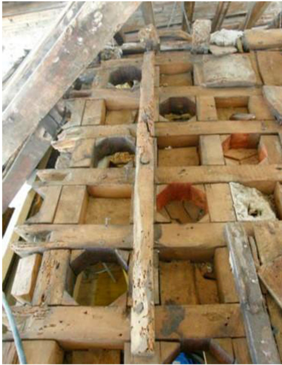
Fig. 18 External side of the almizate . Regular pattern of alternate octagons supporting the eight-point stars (Source: Rodríguez Trobajo 2014)
