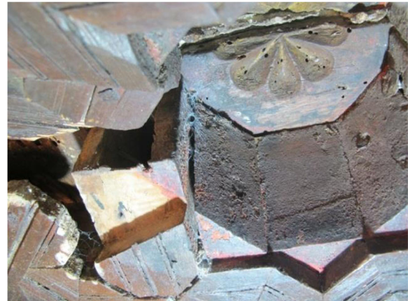
Fig. 13 Disassembled eight-point star on the encounter between the almizate and one slope (Source: Artyco 2015)
