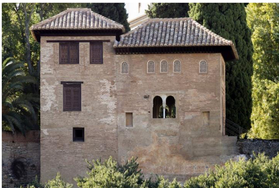
Fig. 4 North-eastern elevation of the Oratory and the House of Astasio, both built over earlier defensive walls (Source: Artyco 2015)
