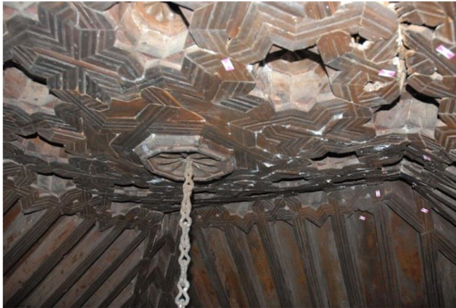
Fig. 12 Profound warping in the upper horizontal plane of the decorated timber framework, the almizate (Source: the author)
