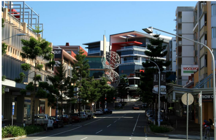
Fig. 7 Façade design and compact development
