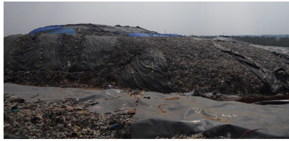
Fig. 2 Waste covered with HDPE geomembrane sheets in landfill site
