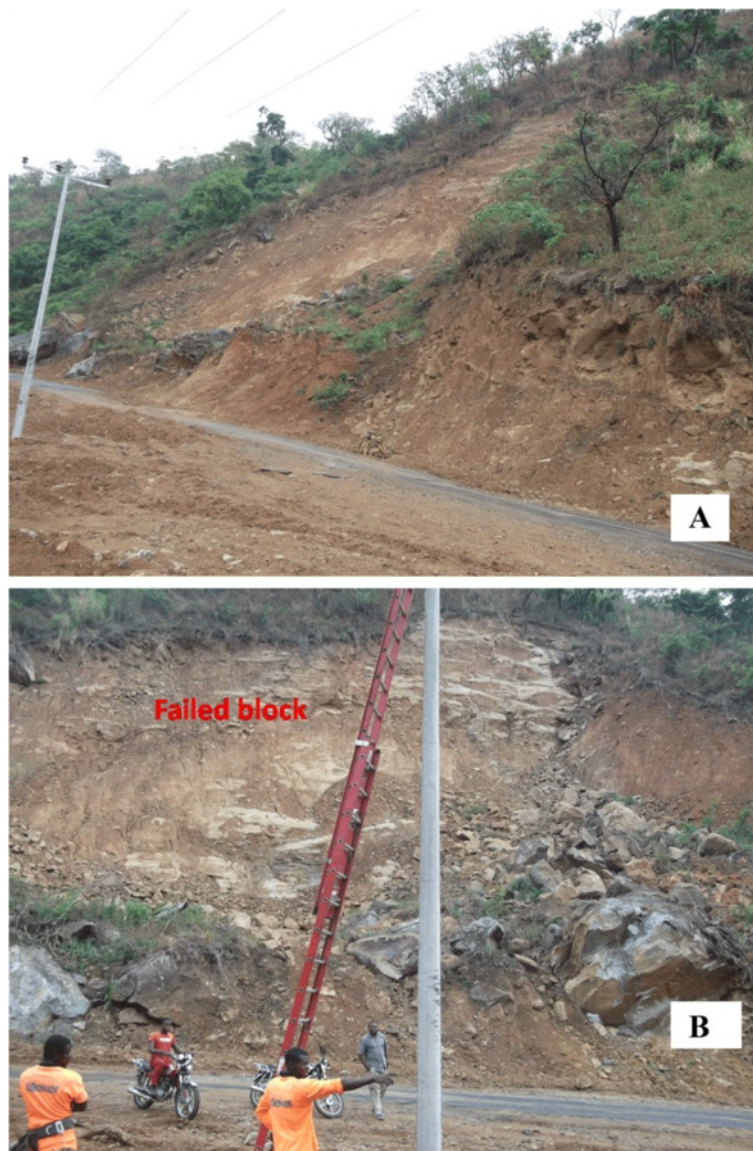
Figure 9 The landslide debris initially covered the road before being cleared in (A) and damaged power cables prompting the erection of a new power line in (B) (photo by Igwe).
