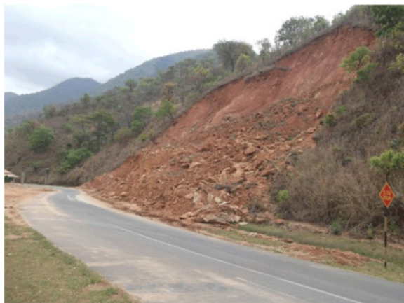
Figure 4 A landslide on the metamorphic terrain in Obudu Calabar (photo by Igwe).
