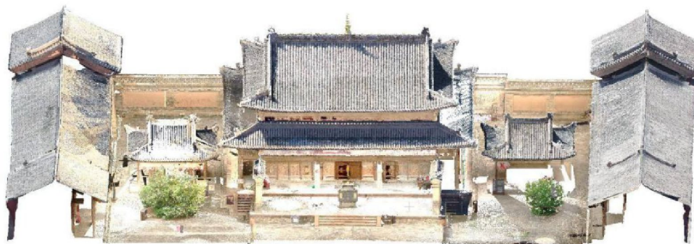
(a) A fully structured Color point cloud of Baoguang building
