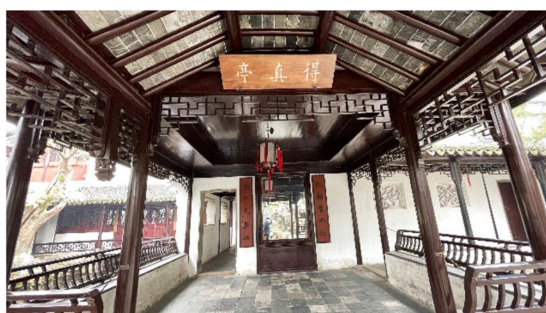
(1) Shedthin tile on the roof of Truth Ting in Humble Administrator's Garden
