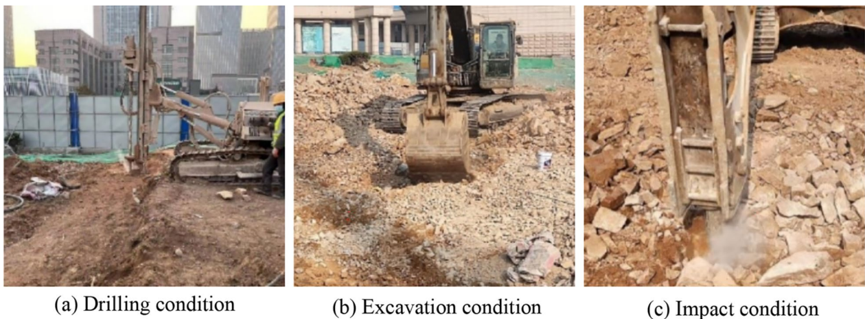
Fig. 5 Construction site of each working condition
