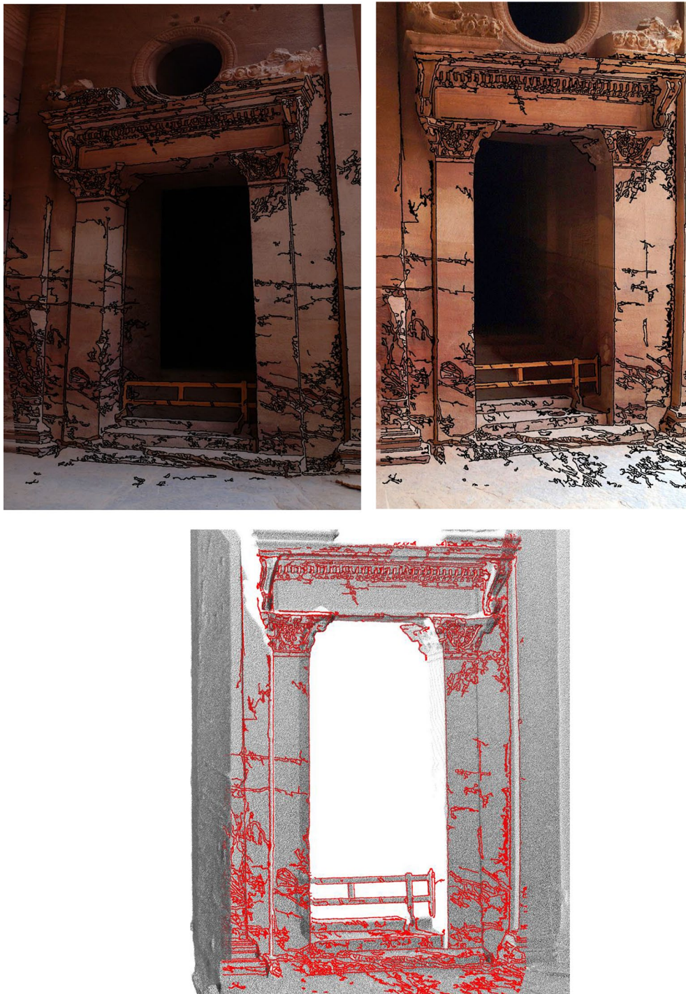
Fig. 11 Mapping the 3D features on different RGB images and the meshed laser model
