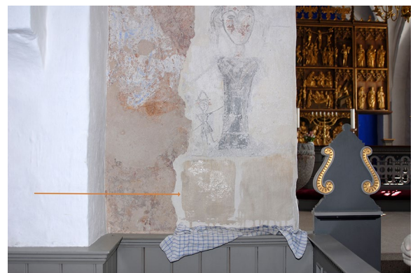
Fig. 5 The lime washed walls of the medieval Nr. Broby Church on Funen, Denmark. The sampling site is below the medieval murals (indicated by the orange arrow ) (Photo: Kaare Lund Rasmussen)
