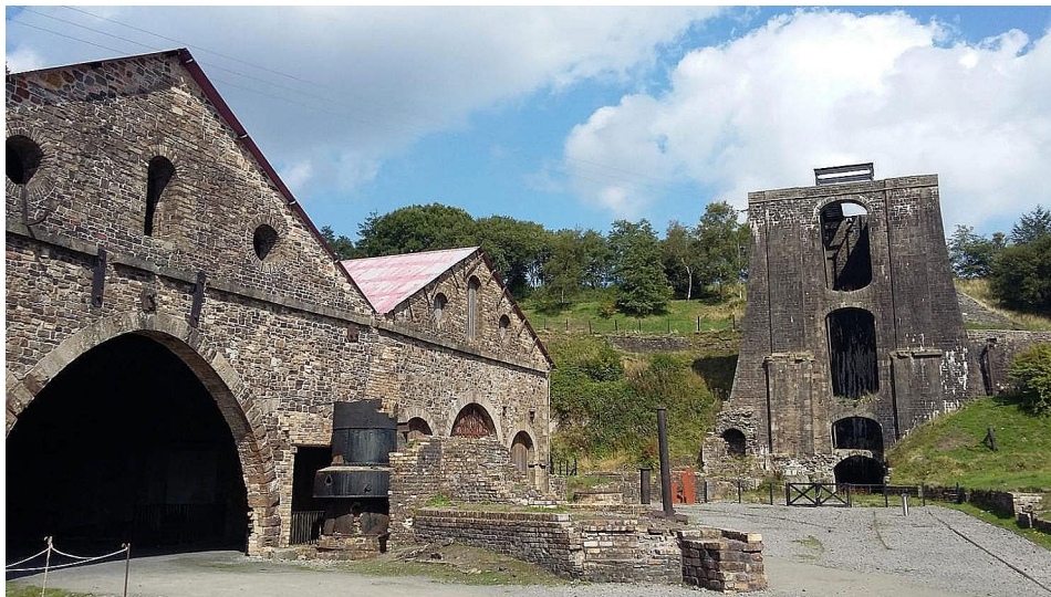
Fig. 1 Ironworks, Blaenavon, Wales (United Kingdom)
