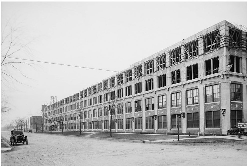
Fig. 1 Packard Automobile Plant, Detroit, Michigan. Architect: Albert Kahn (Photo by unknown author)
