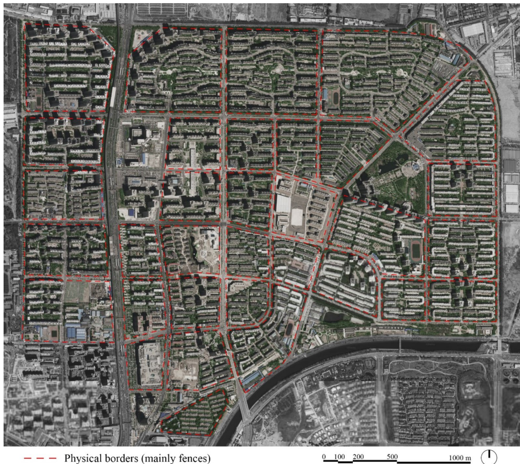
Fig. 6 Plan of the residential district of Tiantongyuan, Beijing. Almost all residential blocks are gated and surrounded by fences (Illustrated by the author based on Baidu maps, 2019)
