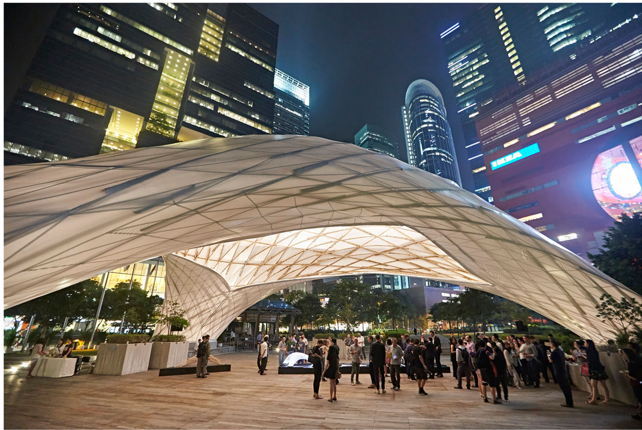
Fig. 2 'ZCB Bamboo Pavilion' during a night-time event
