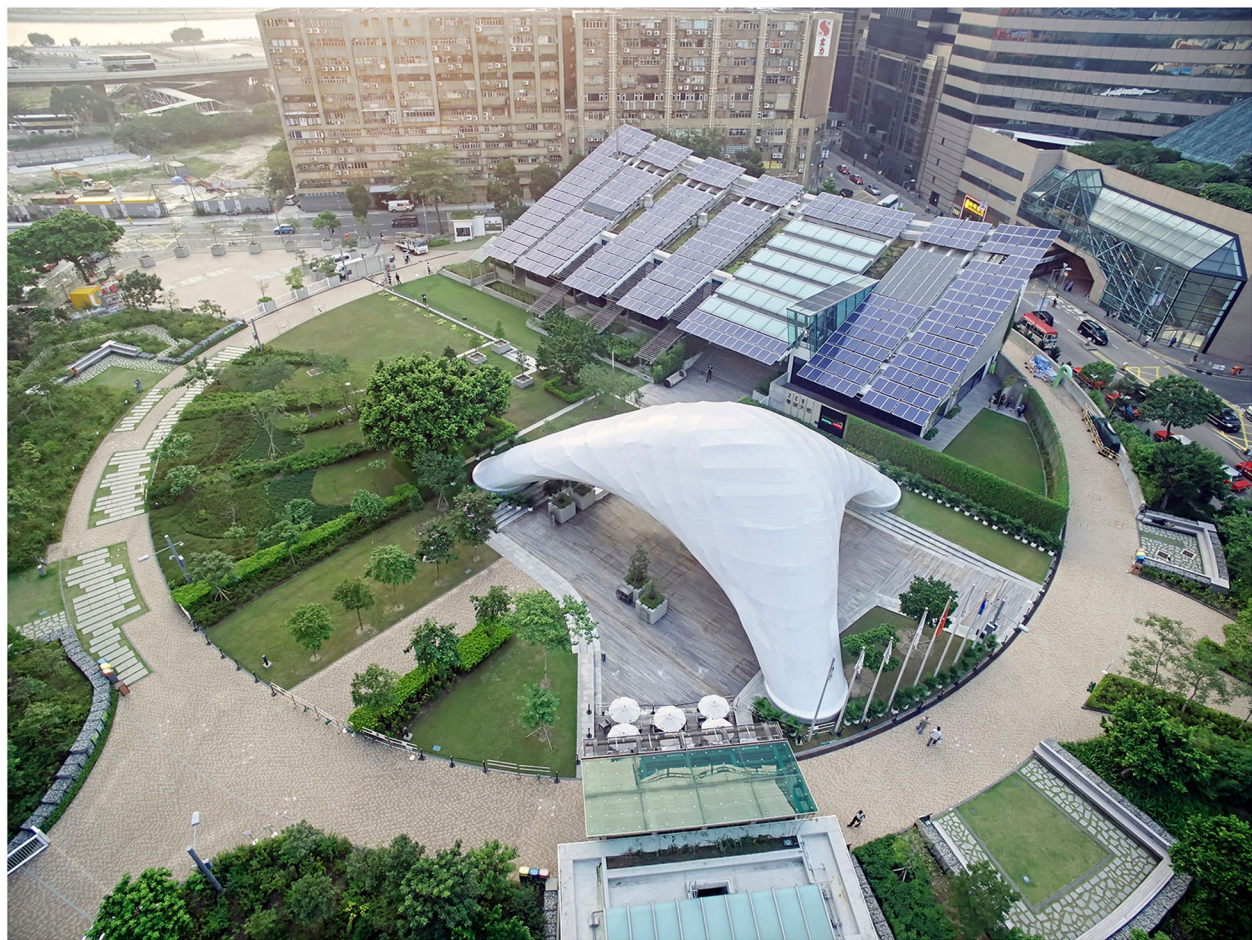
Fig. 19 Aerial view of 'ZCB Bamboo Pavilion' by day
