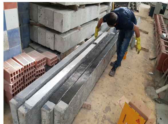
Fig. 4 Attaching the FRP layers on bottom surface of studied beams.
