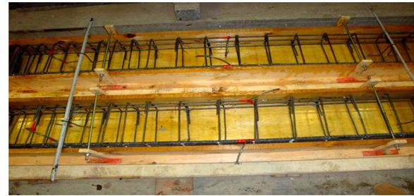
Fig. 3 Steel reinforcement of specimens in formwork.
