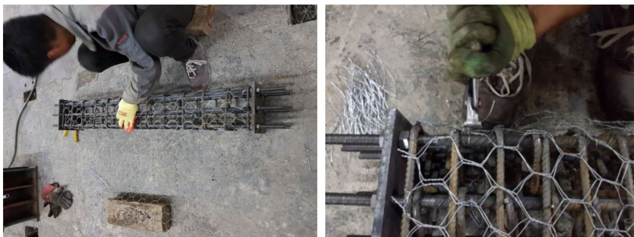
Fig. 3 Fabrication of RC columns confined by HCWM.
