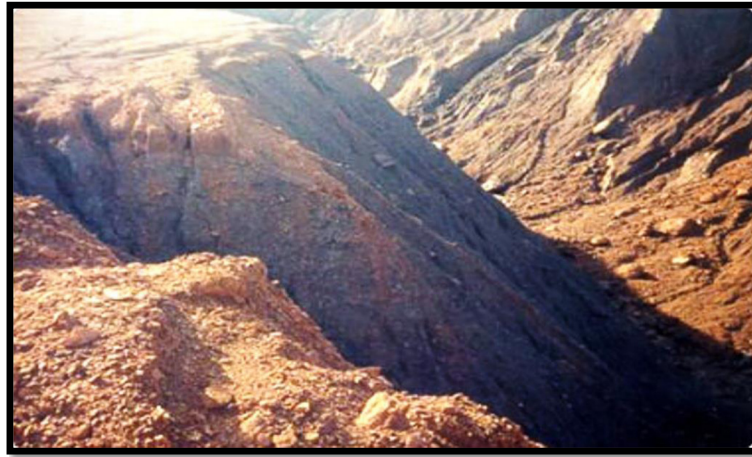
Fig. 3 Slope failure in a waste dump of iron ore mines
