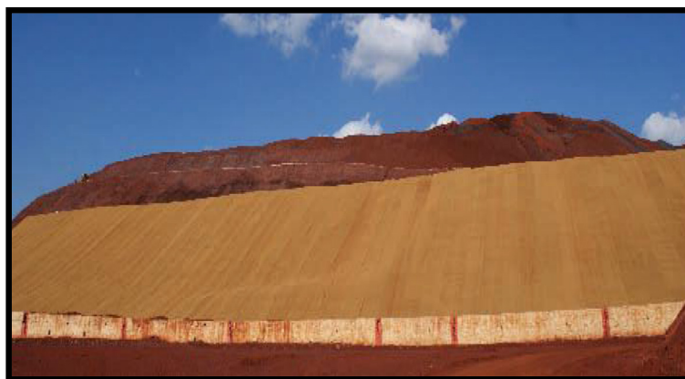
Fig. 4 Installation of coir mat in iron ore mines
