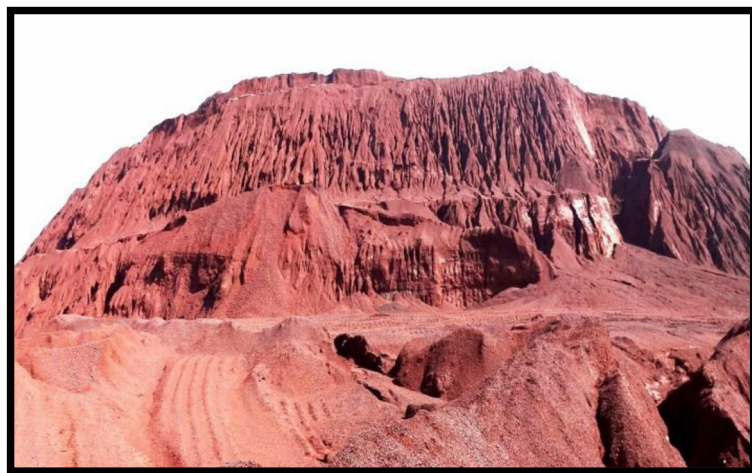
Fig. 2 Slope failure in a fine dump of iron ore mines
