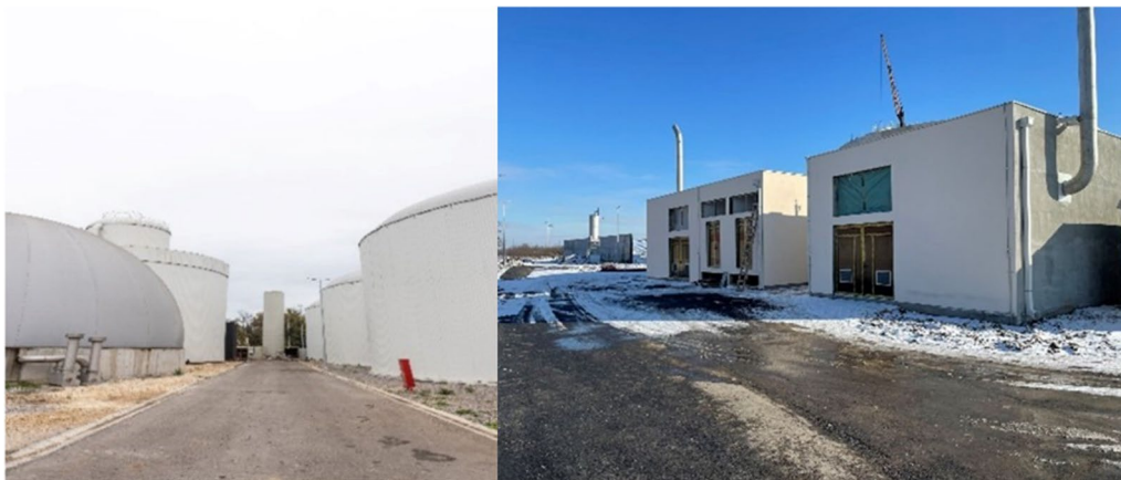
Fig. 1 Biogas plant in Vrbas, Republic of Serbia [61]
