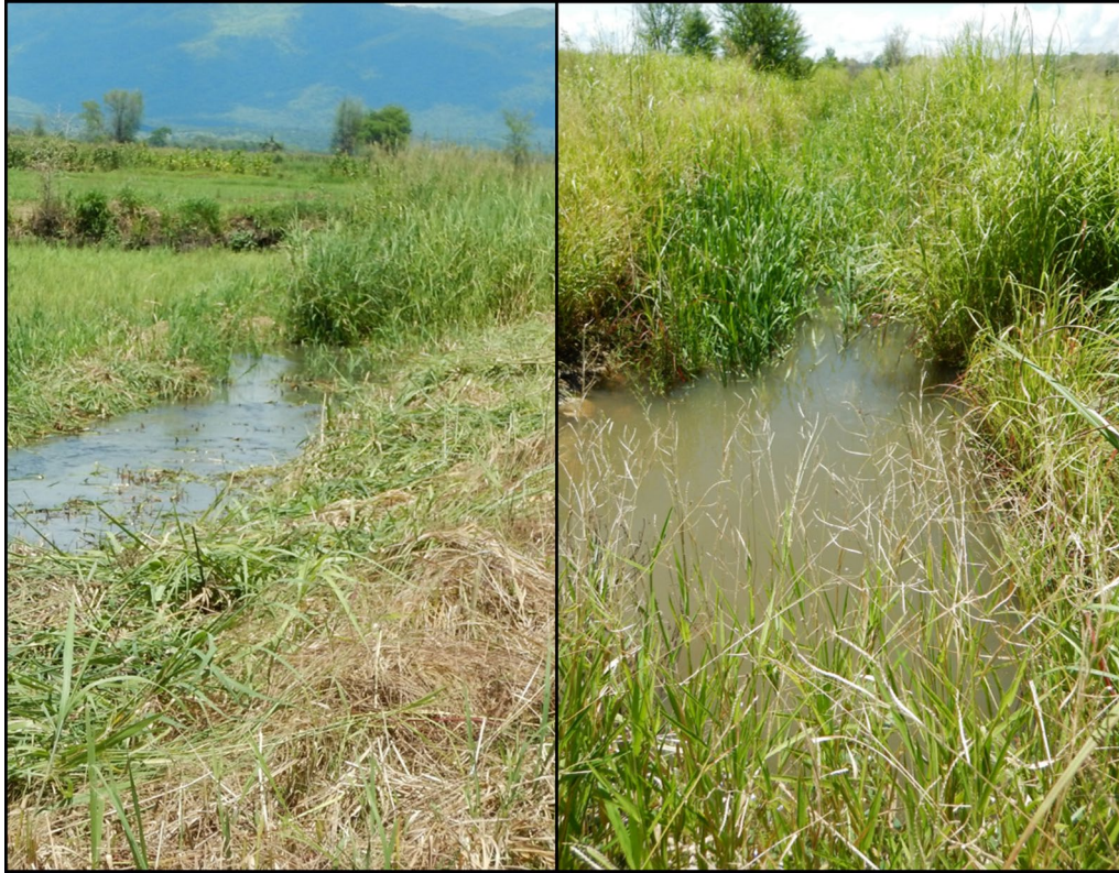
Fig. 10 Evidence of improper maintenance of surface drains; the growth of tall grasses chokes drainage canals preventing proper redistribution of water resources across the scheme
