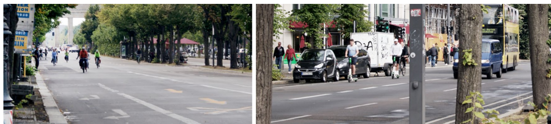
Fig. 8 Site B4 – Berlin, Unter den Linden (south and north); length of observation area: 80 m each; road width: 6.6-m bus lane (south), 3.9-m bus lane (north) and 2.8-m parking lane (north); sidewalk width: 4.2 m (south); 3.4 m (north); pedestrians per 5 min: 41; cyclists per 5 min: 17
