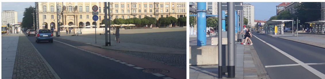
Fig. 5 Site D1 – Dresden, Kulturpalast south and north; length of observation area: 70 m each; on-road bike lane width: 1.6 m; sidewalk width: 6.3 m (north), 3.7-m opening into a 4.1-m pedestrian area (south); pedestrians per 5 min: 35; cyclists per 5 min: 9
