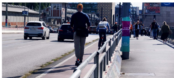
Fig. 3 Site B1 – Berlin, Warschauer Brücke west; length of observation area: 80 m; off-road bike lane width: 1.7 m; sidewalk width: 3.6 m; pedestrians per 5 min: 50; cyclists per 5 min: 41
