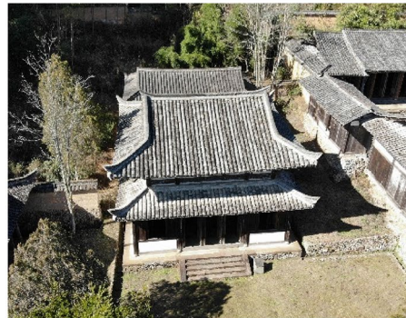
d. Shisi Temple (Built in 1140; Located in China; A representative traditional timber building of Song dynasty)
