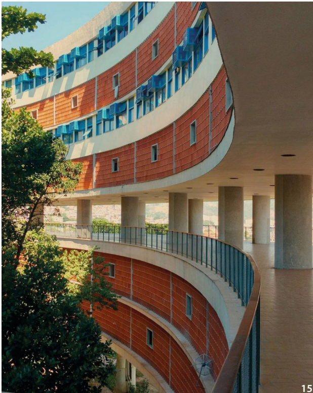
Figure 14 Affonso Eduardo Reidy, Museum of Modern Art, second floor with ducts (Source: Leonardo Finotti).
