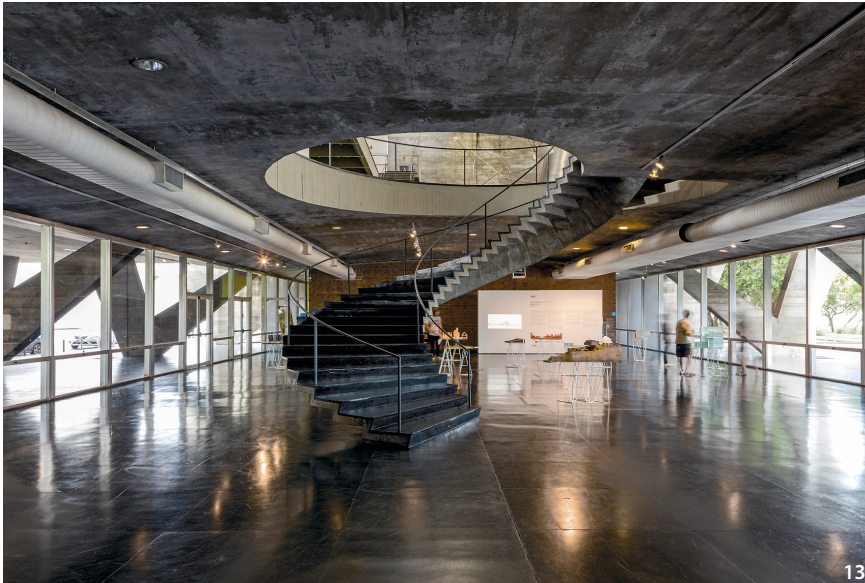
Figure 13 Affonso Eduardo Reidy, Museum of Modern Art, ground floor with ducts (Source: Leonardo Finotti).
