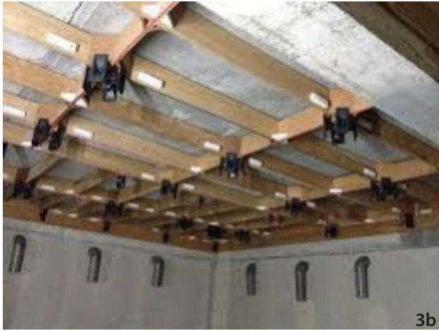
Figure 3b View of alterations and environmental changes made to historic shop-houses for use as swiftlet farms (Source: Archaeological Assessments Ltd.).
