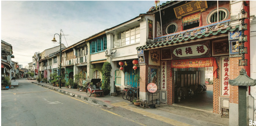
Figure 3a Shop-houses and the built environment that characterises the World Heritage property of Melaka and George Town: Historic Cities of the Straits of Malacca (Source: the author).
