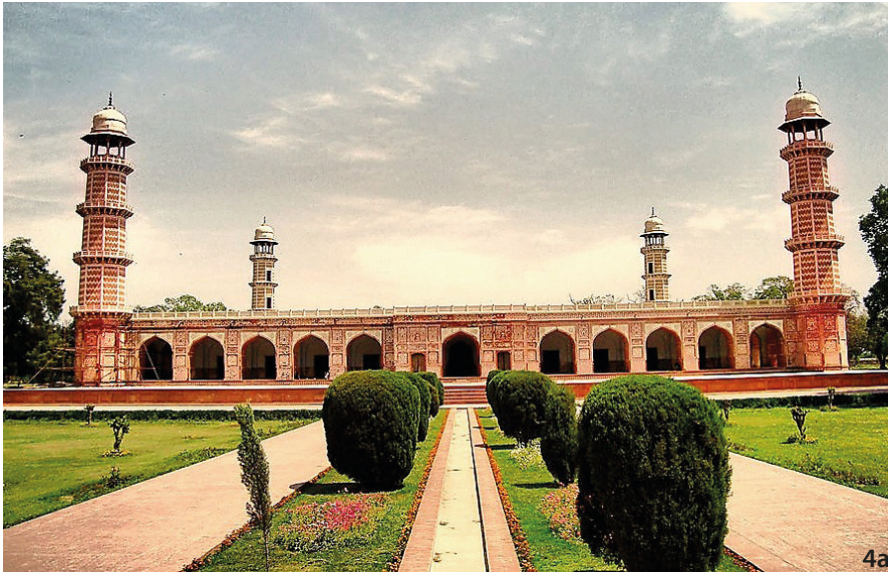
Figure 4a View of the Jahangir's Tomb, part of the World Heritage Tentative List property at Shahdara, Lahore (Source: the author).
