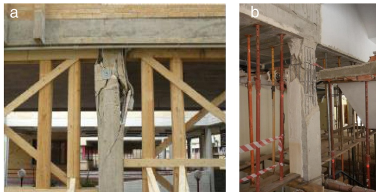
Figure 1 Flexural deficient behaviour in RC columns. (a) In the San Salvatore Hospital, in the 2009 earthquake in L'Aquila, Italy; (b) in a residential building, in the 2011 earthquake in Lorca, Spain.
