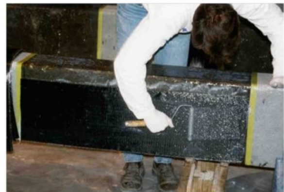
Figure 4 Application of CFRP sheet for Beam-0°/90°, test 1.
