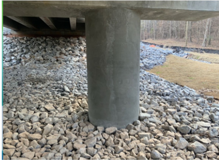
Fig. 3 Riprap protection on bridge pier
