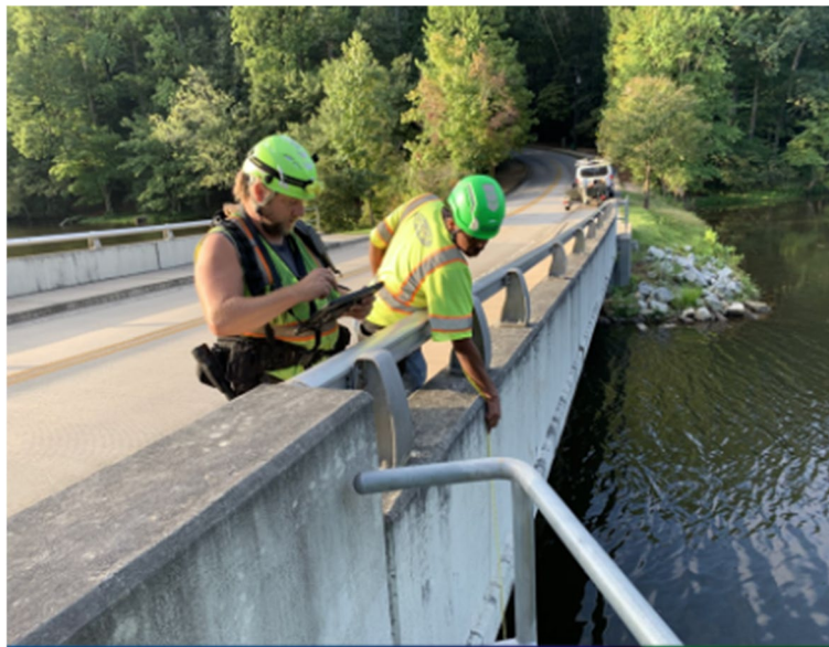
Fig. 4 Visual Bridge Inspection for structural damage
