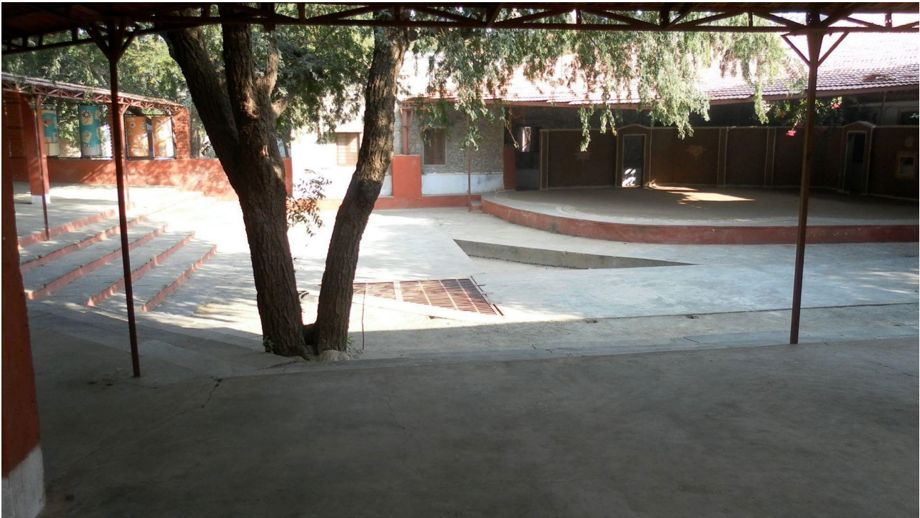
Fig. 9 Water conservation is built into the architectural design of the school (courtesy, Jennifer Patterson)
