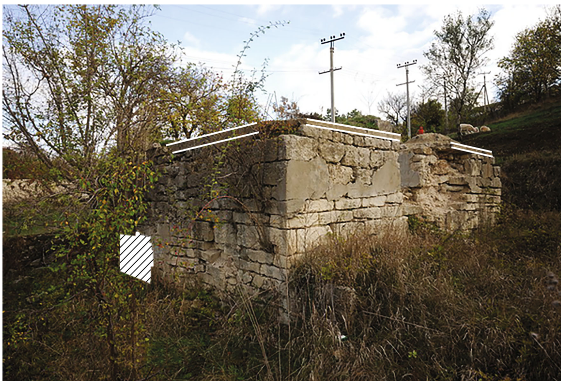
Fig. 3. Hansaray. Eastern structure of presumed Sahib Giray Divan Hall (northern wall) before loss of cladding of well-processed stone (after (Gaivoronskii, 2015)). Black shading on white background shows sub-rectangular entrance to building on northern face of structure. Concrete ceiling slabs are indicated by white lines.
