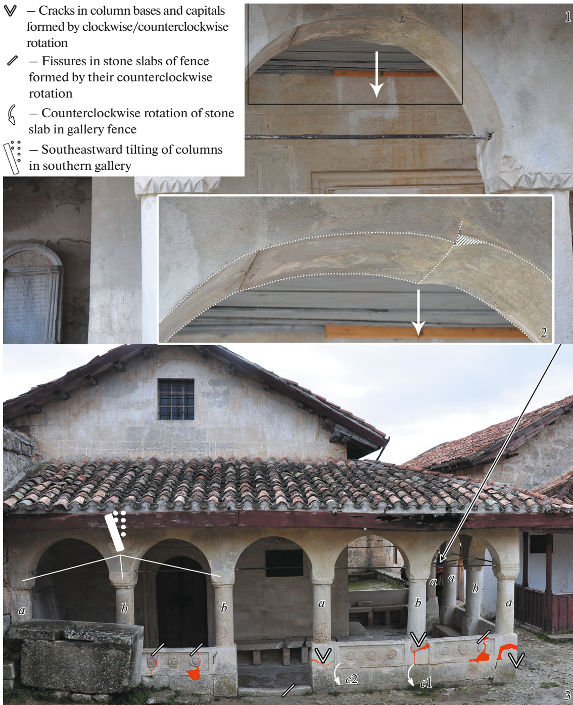
Fig. 9. Chufut-Kale Fortress. Big Kenassa: 1, southwestern gallery with strike 95°; 2, same, close-up view; 3, view of northeastern gallery (red filling shows fissures formed in column bases and fence stone slabs by their counterclockwise rotation): a , columns with stalactite echini on capitals; b , columns with echinus in form of round pillows and octagonal necks; c1 , counterclockwise rotation of column base by 4° in gallery; c2 , counterclockwise rotation of stone slab in gallery fence by 5°.
