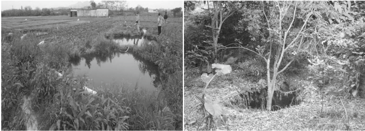
Fig. 1. Two photographs showing typical collapse sinkholes caused by groundwater pumping in the Guanghua basin.
