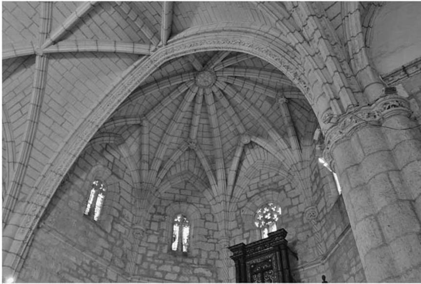
Figure 4: Vaulting in the sanctuary apse, Cathedral of Santo Domingo. Source: Peter Hess.
