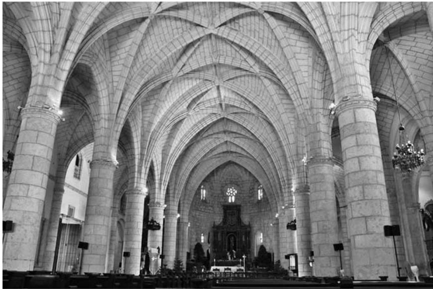
Figure 2: Nave vaulting, cathedral of Santo Domingo. Source: Peter Hess.
