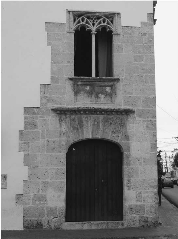
Figure 6: Main entry door, Casa de Tostado (c. 1502), Santo Domingo, Dominican Republic. Source: P. Niell.
