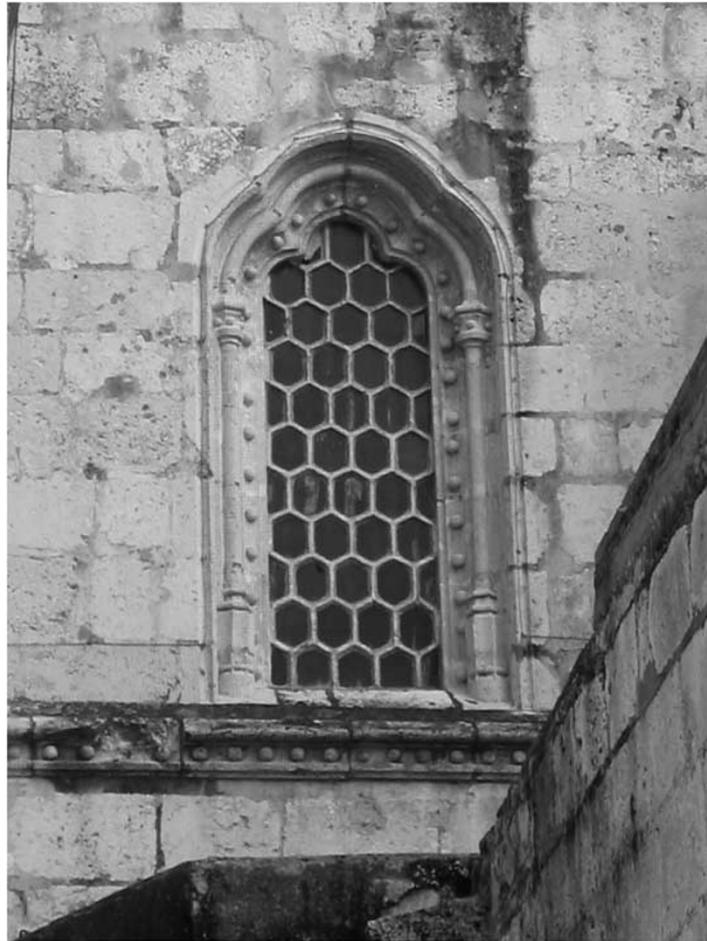
Figure 5: Window from the exterior, Cathedral of Santo Domingo. Source: P. Niell.
