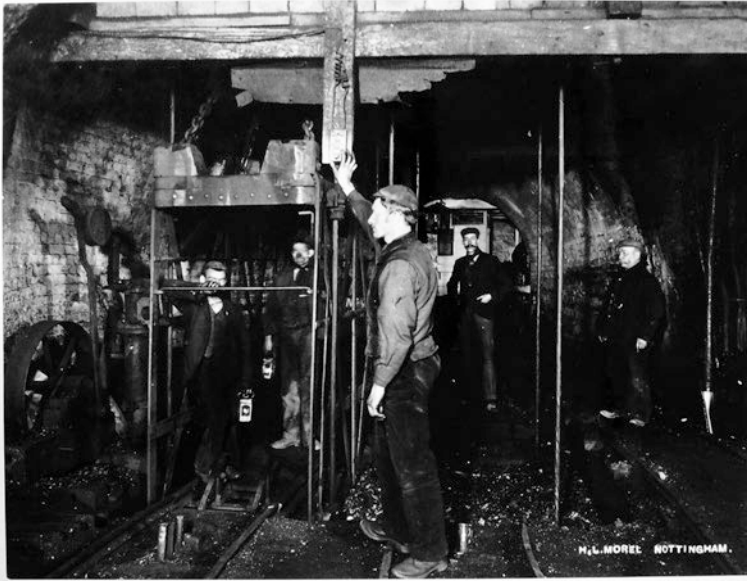
Fig. 10.6 Men ascending in the cage (Reproduced with permission of Local Studies Library, Nottingham)
