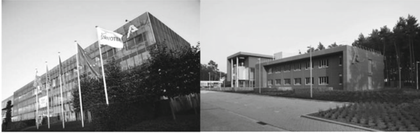
Fig. 13.7 Technology houses of Innotech in Geel and Mol (Belgium)
