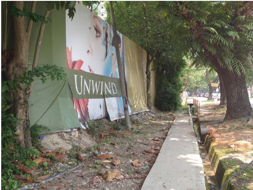
Fig. 7.2 A new residential development in progress in Penang
