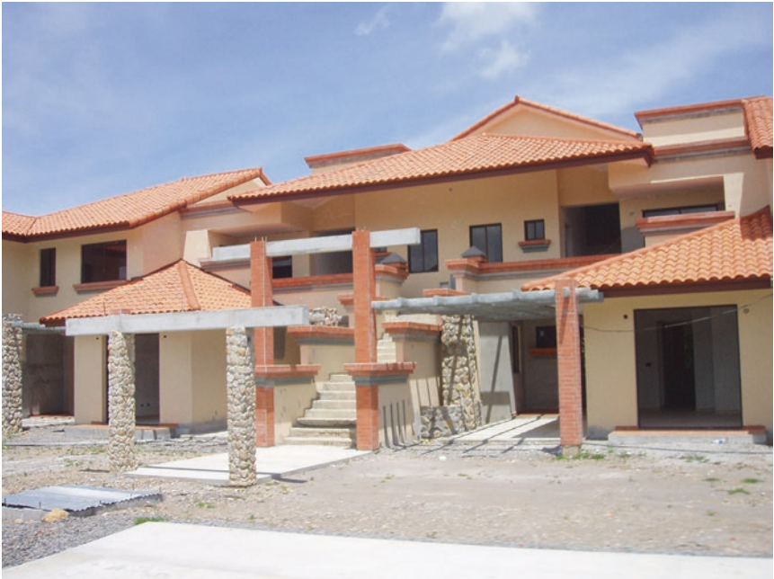
Fig. 7.1 Spanish Villas in Valle Escondido
