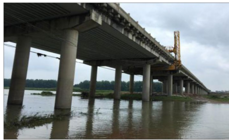
Figure 9. Physical image of bridge.
