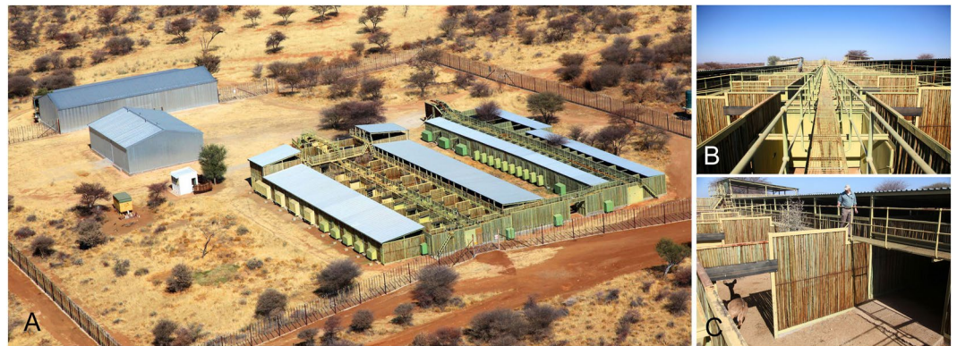
Figure 2. Aerial photograph of the experimental holding facility at the Okosongoro Safari Ranch showing the individual pens as well as the supply buildings and staff quarters (A). To prevent contact with free-roaming wildlife from adjacent areas, the entire experimental holding facility and surrounding area was secured by a single 3.2 m high wire mesh game proofed fence. Overhead catwalks enabled staff to better observe and manipulate animals (B). Individual pen (“boma”) (7 m × 14 m) consisting of a covered - and an open area (C). The sliding door could be used to connect the pen with an adjacent pen for separating single animals. The height of the indoor part of the pen was 3 m and the outdoor section was surrounded by a 3 m high wall.
