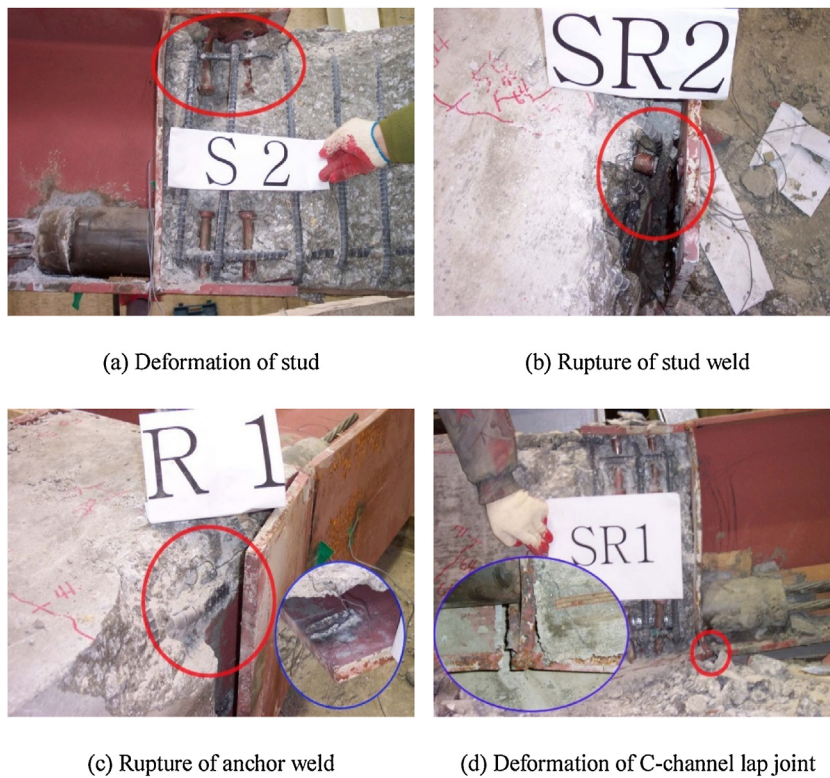
Fig. 11 – Details of failure in steel-concrete connections of hybrid girder test members.
