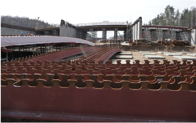
Fig. 3 – Steel beams with continuous shear connectors before application in animal crossing bridge PE4 over S7 expressway in Poland.
