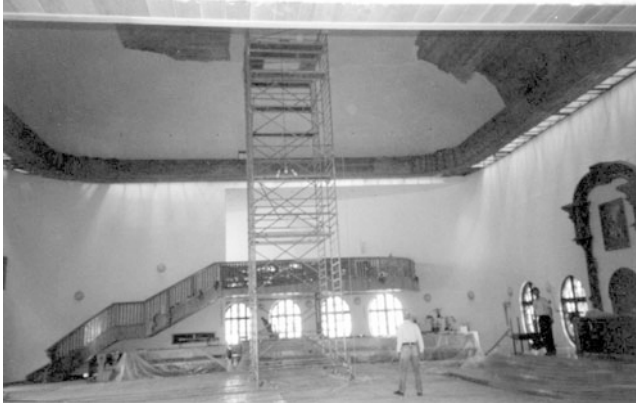
Fig. 30 – Placing of a gypsum finishing coat on the concrete dome surface.
