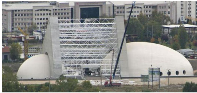
Fig. 11 – Reinforced concrete ellipsoid dome of CSO Concert Hall of up to 2000 concert-goers, Ankara, Turkey [29,30].
