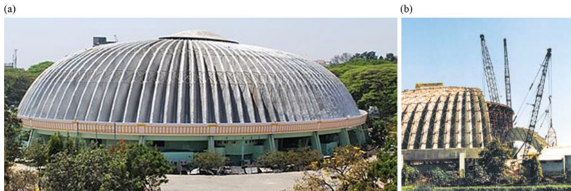
Fig. 9 – Elliptical Sree Kanteerava Indoor Stadium in Bangalore. Capacity 5000, built: 1995, architecture design: Sundaram Consultants (a) Stadium view [27] (photo: Sanyam Bahga), (b) erection of roof elements [28].
