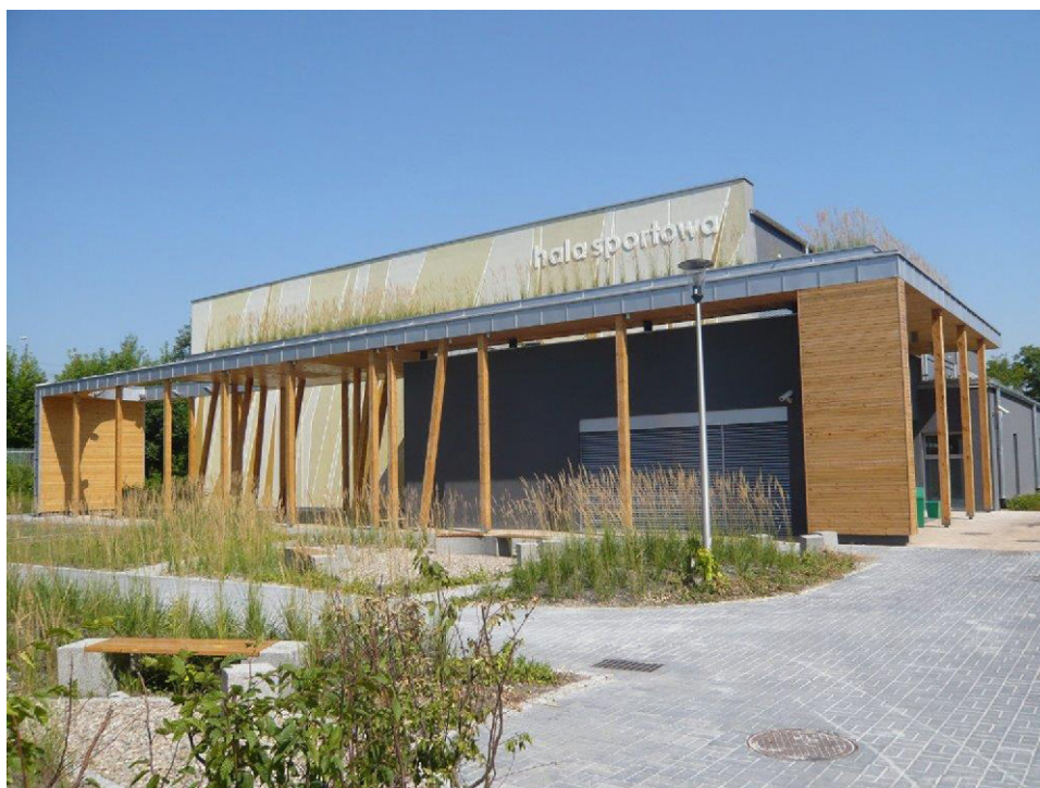
Fig. 1 – South facade of sports hall building.
