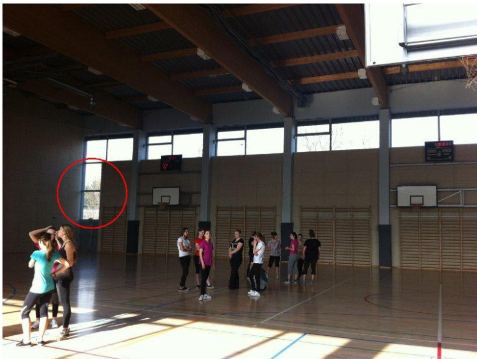
Fig. 4 – Internal view of the west wall with horizontal and vertical strips of glazing.
